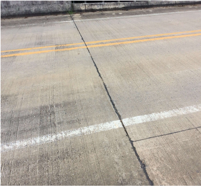
PHOTO 1 Description Joint - Bent 1: Loss of adhesion
