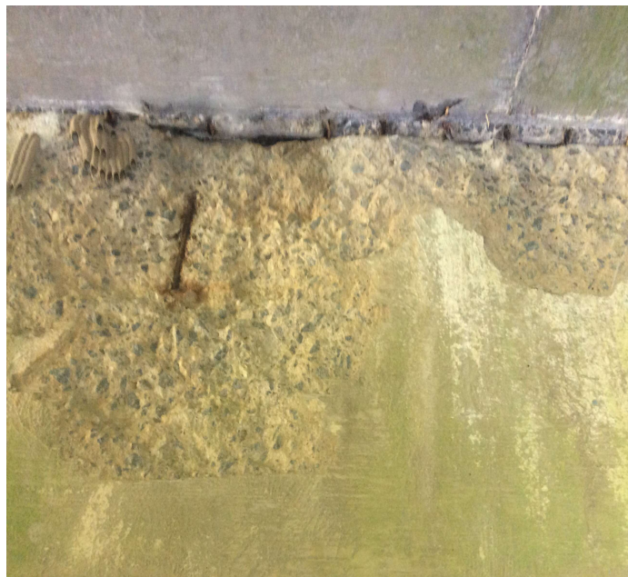
PHOTO 1 Description Bent 3 spalls and spall with exposed rebar.
